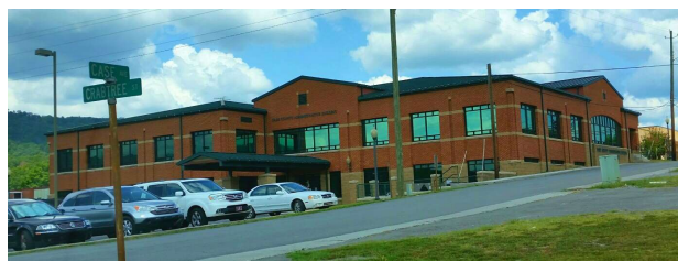
Figure 6. Dade County Administrative Building
