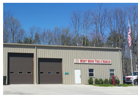
Figure 59. West Brow Fire Station.
